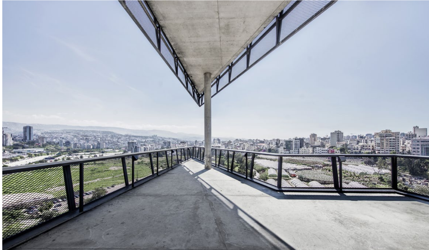
Generous balconies offer impressive views of the city – for now.
